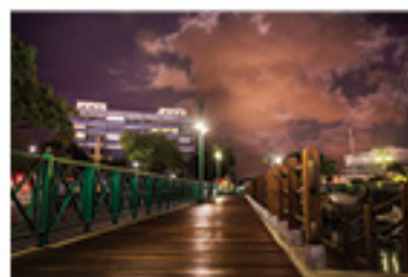
Completed and reopened Wickham Lewis Boardwalk.
